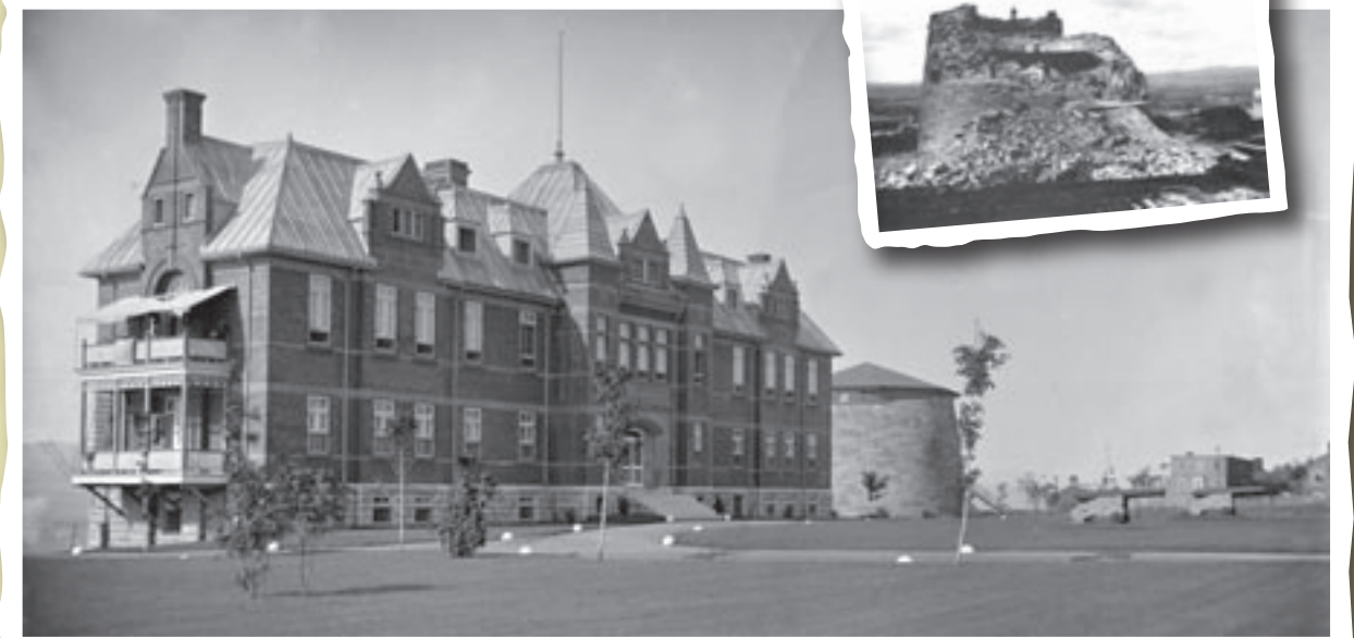
THE FIRST PAVILION OF THE JEFFERY HALE HOSPITAL (PHASE ONE) BUILT ON SAINT-CYRILLE STREET. THE LOT ALSO INCLUDED FARM BUILDINGS AND ONE OF THE MARTELLO TOWERS BUILT IN 1805-10, WHICH WAS DEMOLISHED LATER TO BUILD THE MACKENZIE WING.
