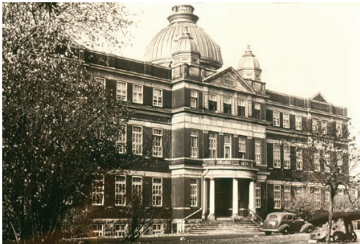
THE MACKENZIE MEMORIAL BUILDING. THIS NEW WING (PHASE TWO) WAS INAUGURATED IN 1906.
